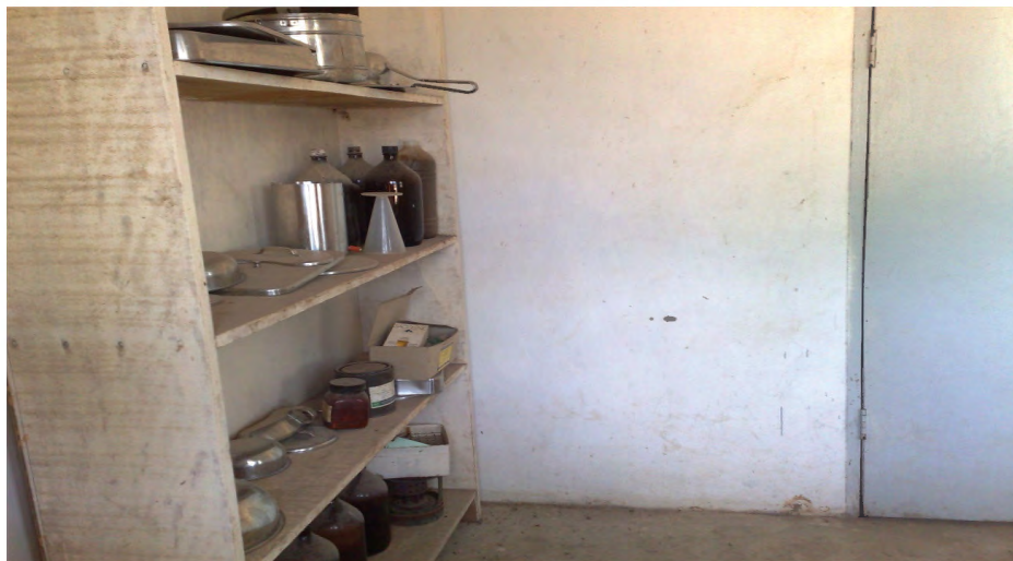
Figure 6: Abandoned Store at the Health Centre.
